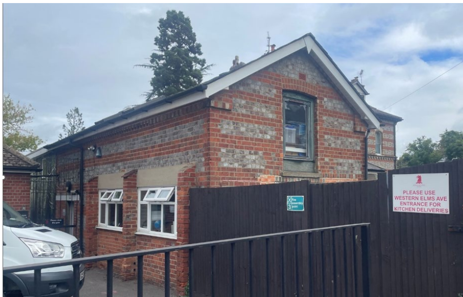
Image of the former Coach House of No. 62 within St Edward's Prep School at 64 Tilehurst Road
