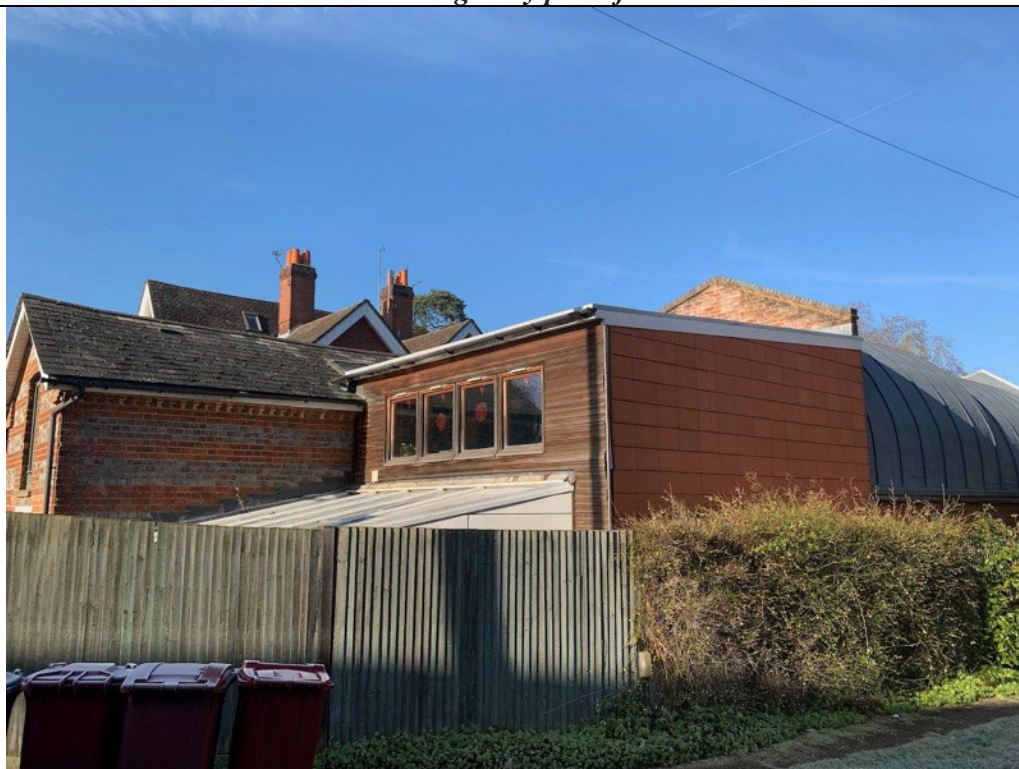
Coach house from the street in front of 62 Tilehurst Road. Note the extension between the building and the boundary, there are also extensions to the rear.
