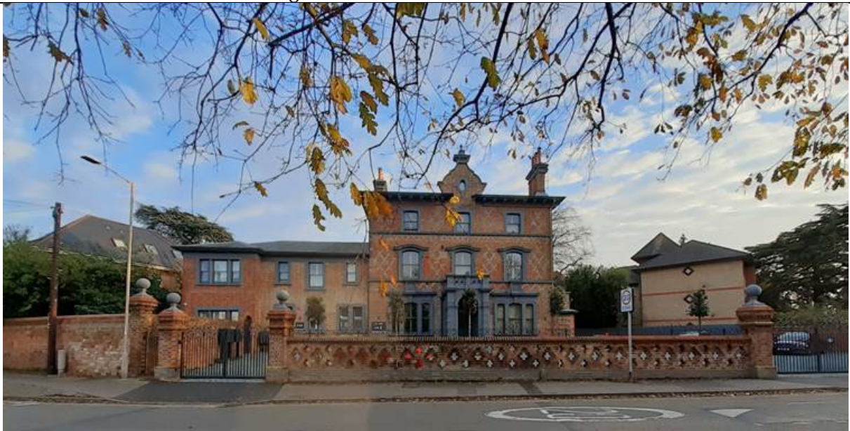
24 Southcote Road (1865) in December 2022 following refurbishment from the west.
